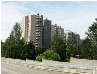
View of first towers from McInnes Overpass 2016.
