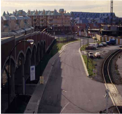
View from McInnes overpass, 1987. (NWMA IHP9563-0654)
