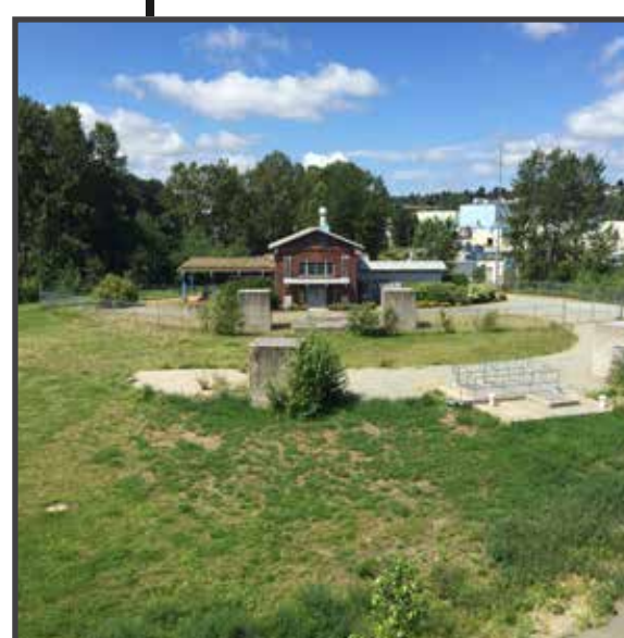
Metro Vancouver Wastewater Storage Facility
