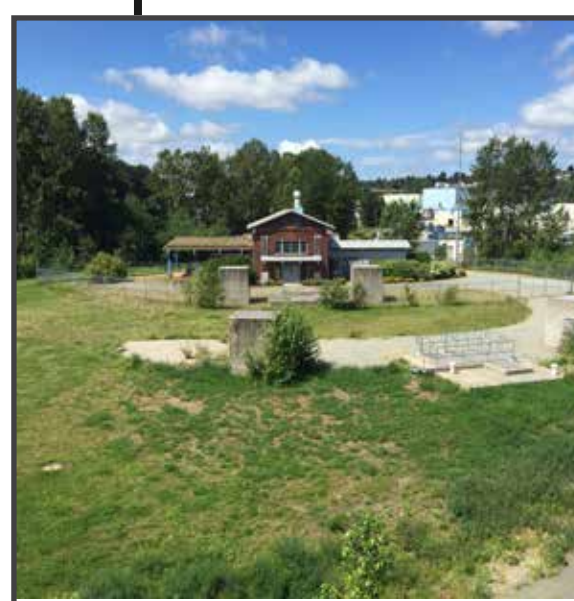
Metro Vancouver Wastewater Storage Facility
